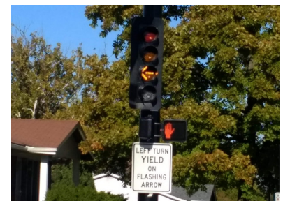
Flashing Yellow Arrow Phases 1 and 2 City of St. Charles, MO
