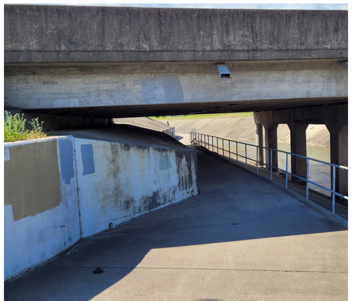
Figure 5.22 - Routine maintenance also includes covering up graffiti and repainting walls.
