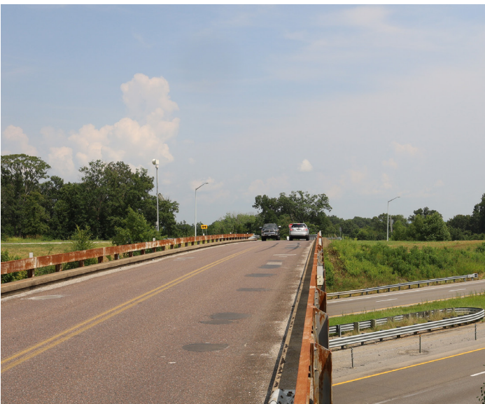
Figure 4.18 - Image of Hopper Rd (County Rd 314) & Hwy 55 crossing
