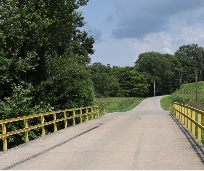
Figure 4.19 - Image of Country Road 318 bridge over Williams Creek
