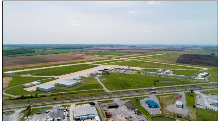
Figure 47: Cape Girardeau (CGI) Regional Airport
